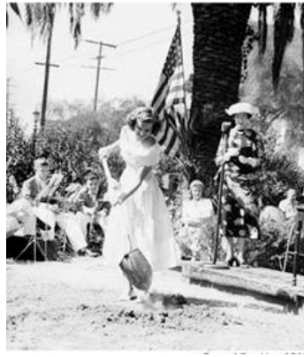
Ground Breaking Day
